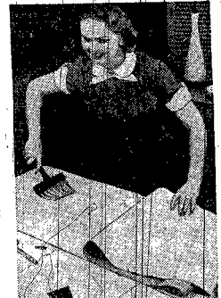
Step 1: Cut strips, 16 inches longer than height of wall. Unroll one strip at a time and brush on paste. Lift up both ends and fold over to center of strip. Now wallpaper is ready to hang.
